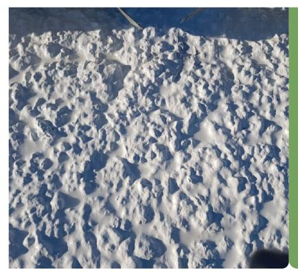
Even where the embedded gravel was still prominent, the end coating of Weatherskin has immersed it under a tough blanket that can be walked on and easily serviced without causing any problems. The Weatherskin team will re-visit this roof every year it is warrantied to protect the client and their investment.
