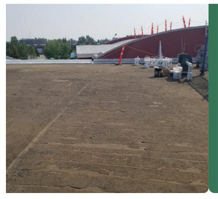
Weatherskin came to the rescue, removing as much of the gravel as possible. The remaining embedded gravel would stay behind. First, all the terminations, scuppers and perimeters were properly sealed and protected with high tensile fabric interlaced into the first 2 coats of the Weatherskin membrane
