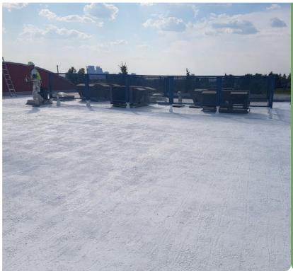
Any seams in the tar paper that have the potential to become trouble areas or deficiencies later were sprayed first to ensure they would be completely sealed by the basecoats. Even a single void in the coating can cause issues later, but they are easy to spot when you're applying light grey over a black substrate.
